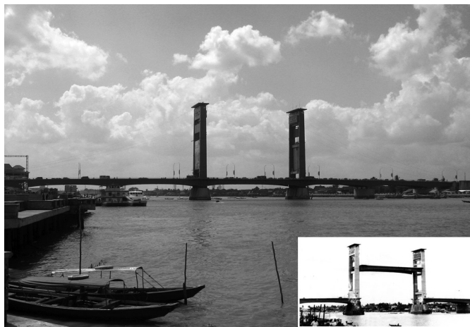
FIGURE 21.39 Ampera's main bridge (inset: the lifting of the central span).
