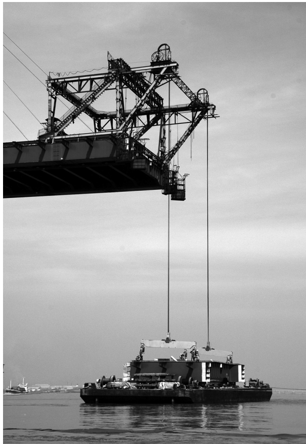
FIGURE 21.106 Typical erection of the steel box girder segments.
