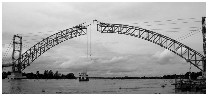
FIGURE 21.62 Erection of the main span of the bridge.
