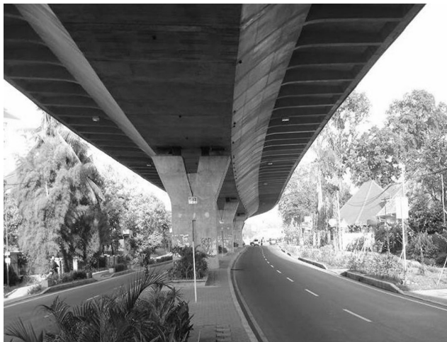
FIGURE 21.72 Precast segmental concrete box girder of the Surapati Viaduct.
