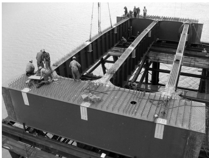
FIGURE 21.104 The segment of the main bridge span after erection.
