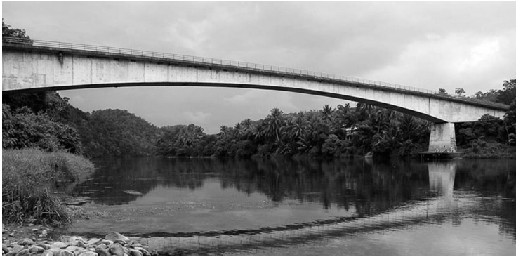
FIGURE 21.29 The Rantau Berangin Bridge (201 m), the first cantilever segmental concrete bridge in Indonesia.
