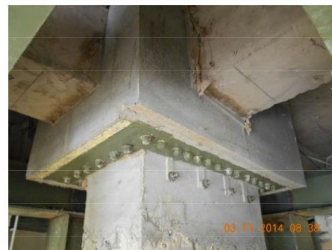
(b) BC enlargement and additional column rebars
