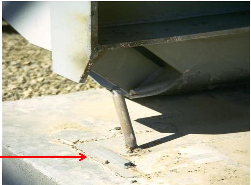
Detail of the failed anchor, rupture at the threaded section of the bolt
