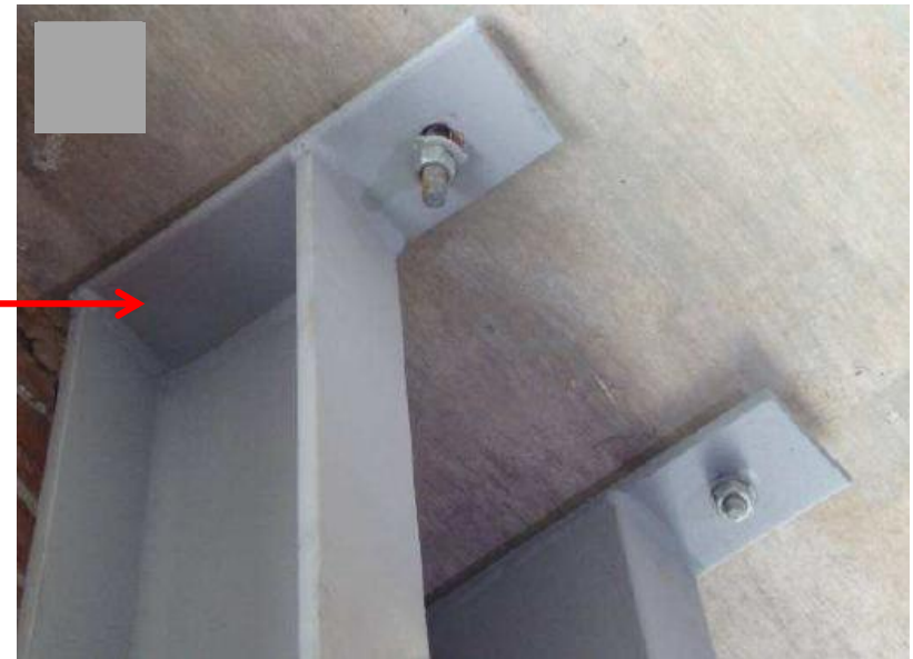
Detail of the displaced anchors at overhead footing of the retrofit steel frame
