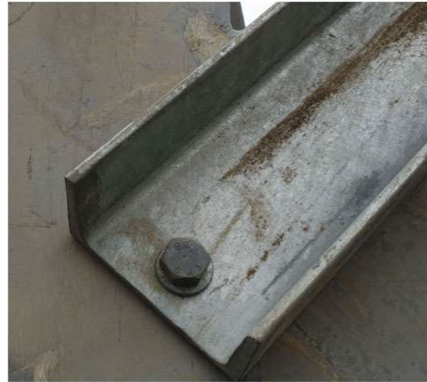
Gambar 53. Detail sambungan bracing (pilon arah tekuk)
