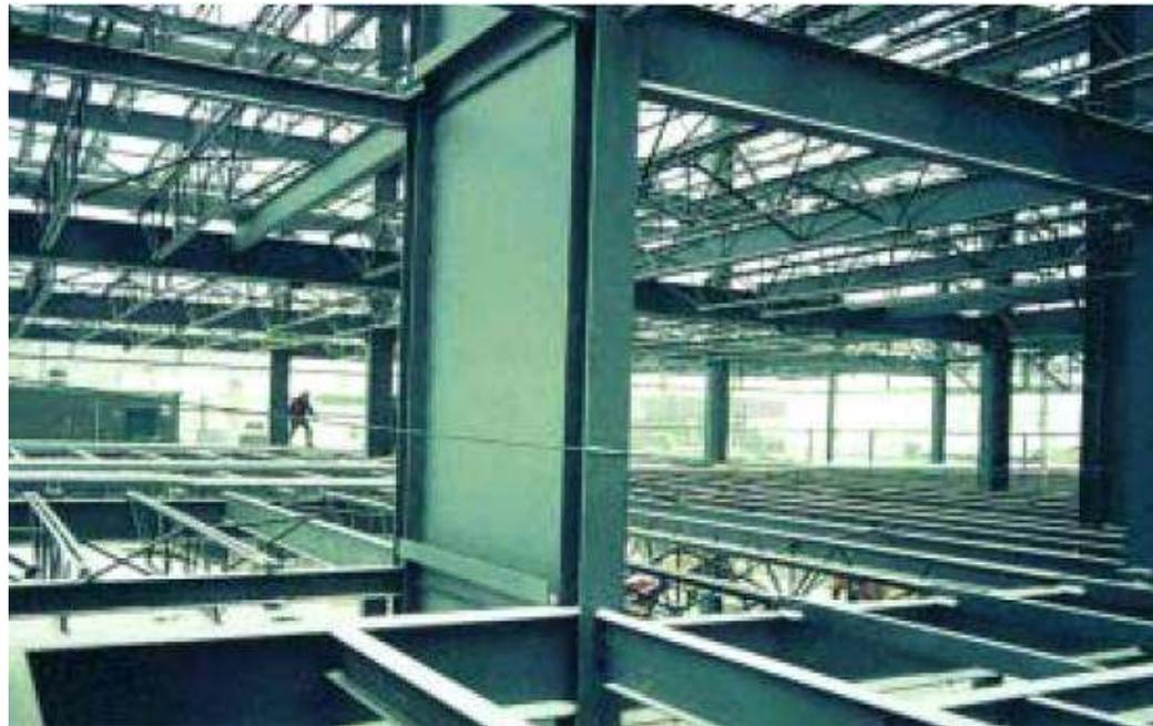
Steel Plate Shear Walls (Seilie and Hooper 2005)
